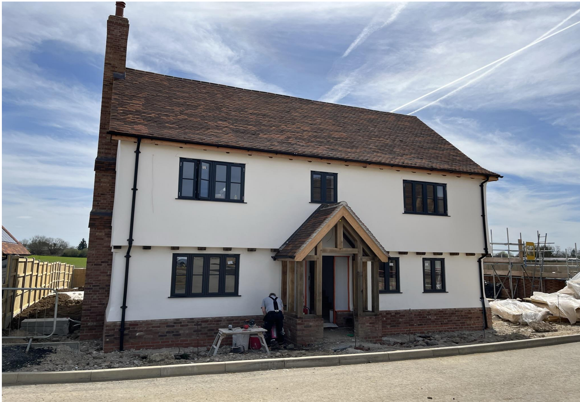
Site Photos – Example of housing palette taken from adjacent Phase 1 site
