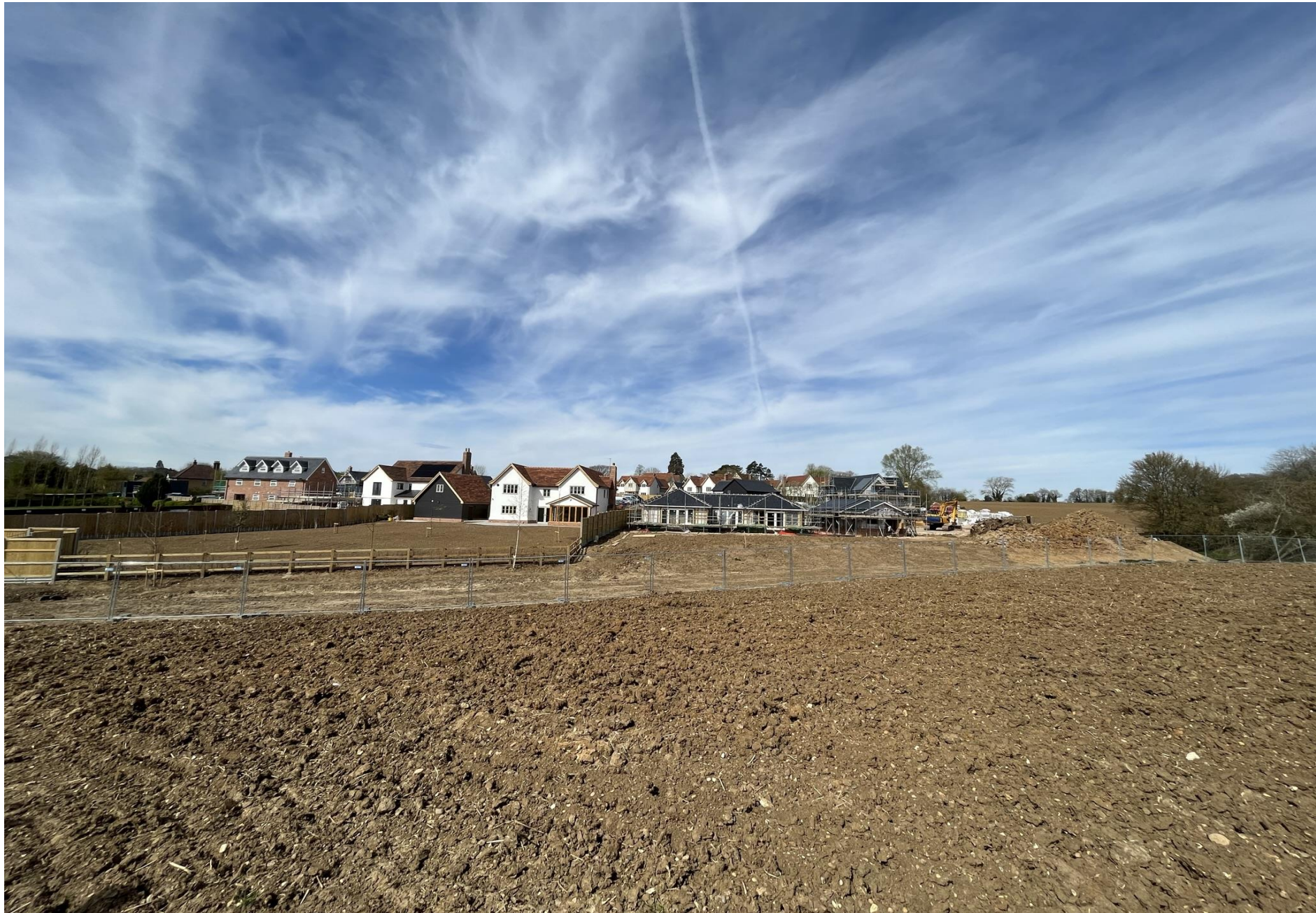
Site Photos – Looking North-West at Phase 1
